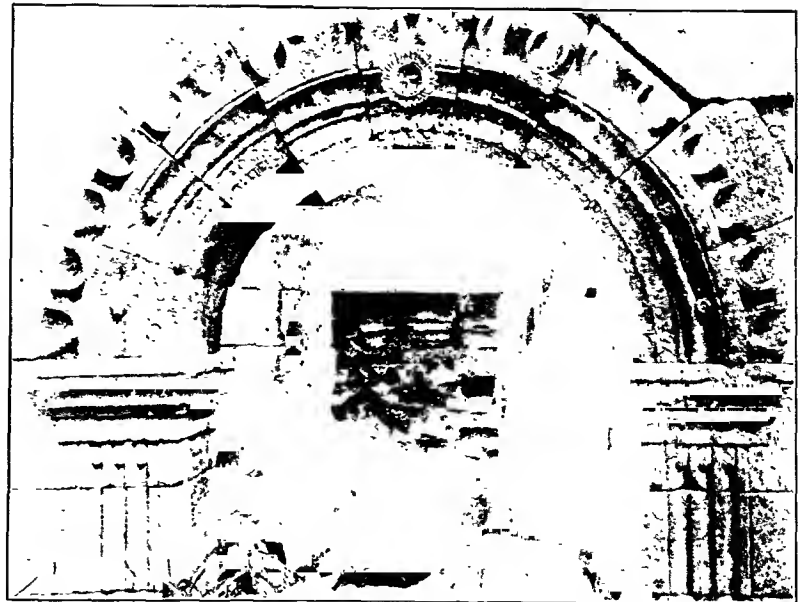
Entrance to a villa at Ruweha.
